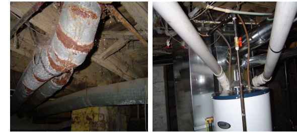
Before and After: Furnace Work
