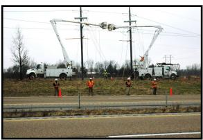
J.F. Electric crew members working on the new Ameren Illinois substation in Collinsville safely pulled power lines across all lanes of Interstates 55-70 to be hooked up to the substation. The substation added capacity to meet increasing customer load growth in the three communities while reinforcing the existing electric system in Madison County and enhance service reliability.
