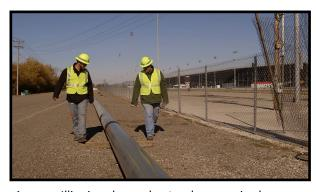
Ameren Illinois enhanced natural gas service by upgrading a high-pressure distribution gas pipe that runs adjacent to Gateway Motorsports Park. The new 12-inch coated steel pipe will fully protect the pipeline from corrosion while allowing for increased system capacity, safety, and reliability to the residential, commercial, and industrial customers served in Madison, East St. Louis and surrounding areas.
